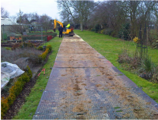
Examples of temporary ground protection mats.
